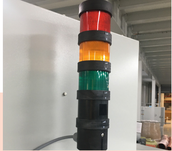
Safety stack light status indicator
