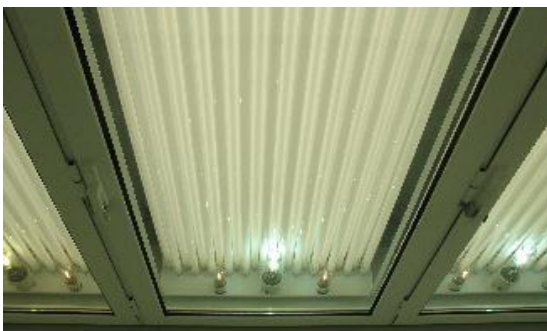
Light canopy composed of HF Fluorescent Tubes, Metal Halide and Halogen bulbs
