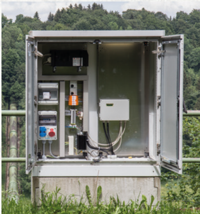
The stationary FLUXUS® ADM 7407 is used as transmitter.
