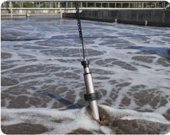
(Sensor holder EH/U 170 in combination with swing mounting assembly EH/F 170-1,5)
